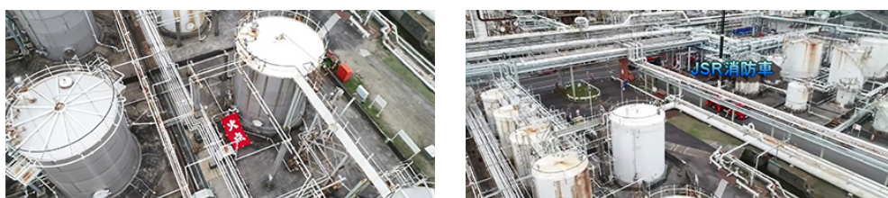
Drill to identify locations of fire with a drone at the JSR Yokkaichi Plant
