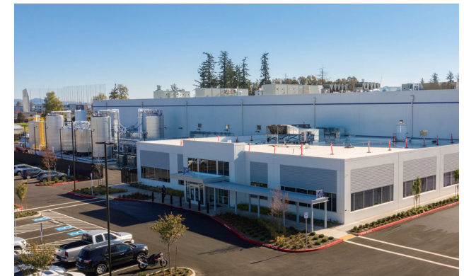
New functional cleaning solutions production facility in the U.S.
