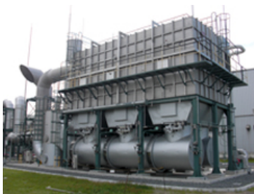
Dried-synthetic rubber waste incinerator (Kashima Plant)
