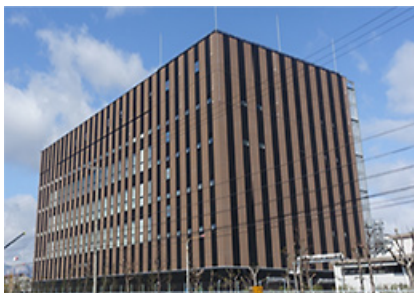
JSR Center of Materials Innovation HAL E-COAT is also used on the Center's roof.
