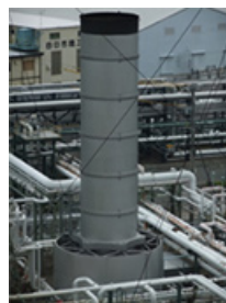
Ground flare (Yokkaichi Plant)
