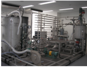
Miniature Plant in Yokkaichi Training Center
