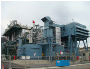
Natural gas-fired turbine cogeneration system (Yokkaichi Plant)
