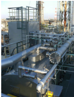
Sludge dryer system (Yokkaichi Plant)
