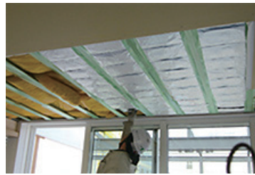
CALGRIP™ being installed in a ceiling
