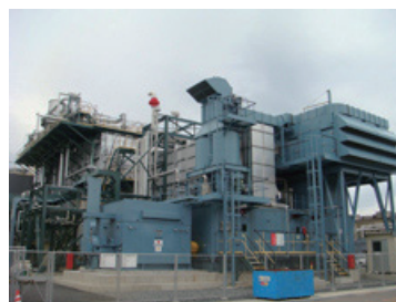
Natural gas-fired turbine cogeneration system (Yokkaichi Plant)
