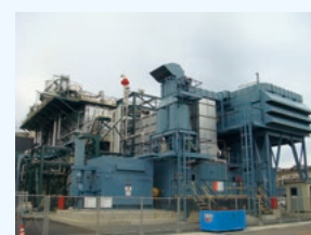
Natural gas-fired turbine cogeneration system (Yokkaichi Plant)
