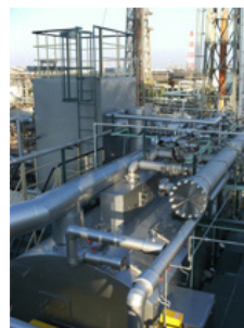
Sludge dryer system (Yokkaichi Plant)
