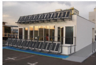
Next-generation housing developed by the University of Tokyo (CALGRIP™ used in ceilings and floors)
