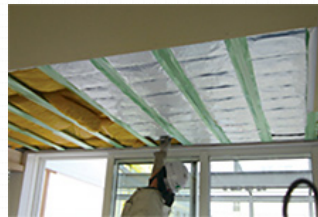
CALGRIP™ being installed in a ceiling
