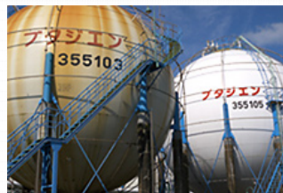
SIFCLEAR™ is used on the right butadiene tank at the Kashima Plant.
