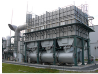
Dried-synthetic rubber waste incinerator (Kashima Plant)
