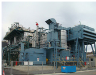
Natural gas-fired turbine cogeneration system (Yokkaichi Plant)
