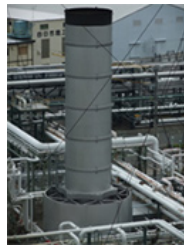
Ground flare (Yokkaichi Plant)
