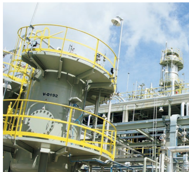
SSBR plant of JSR BST Elastomer, Thailand
