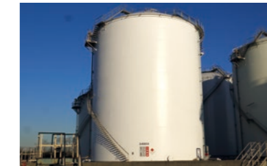
Example of use of antifouling, thermal insulating paint containing SIFCLEAR™ (Cylindrical tank (JSR Kashima Plant))
