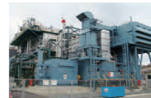
Cogeneration system at Yokkaichi Plant
