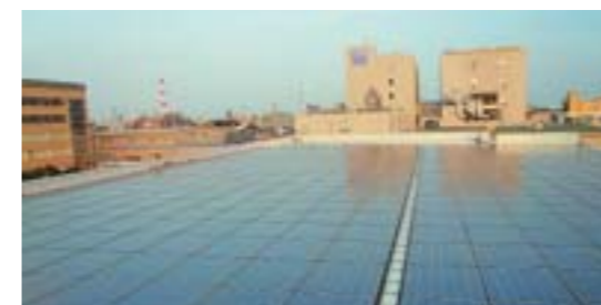
The photovoltaic power generation system installed in the new building
