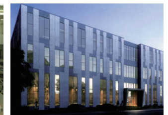
The center is scheduled to start operation in 2022.
