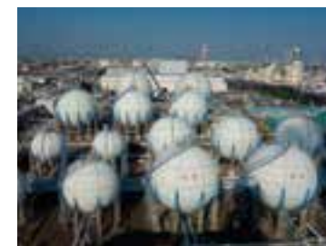
Spherical tanks: Withstands large-scale earthquakes (600 gals)
