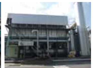
Regenerative thermal oxidizer: Measures against volatile organic compounds and offensive odors
