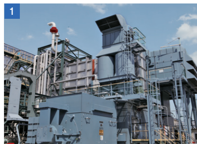
Cogeneration facilities in the Yokkaichi Plant
