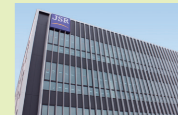
Main administration building of the Yokkaichi Plant. The black parts of the wall have been coated by a SIFCLEAR™-based paint.
