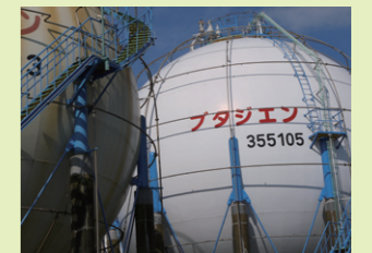
Butadiene tanks in the Kashima Plant. The right tank is coated by a SIFCLEAR™-based paint.
