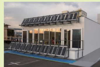
The University of Tokyo's next-generation energy-saving model house (CALGRIP™ was used in the ceiling and floor.)
