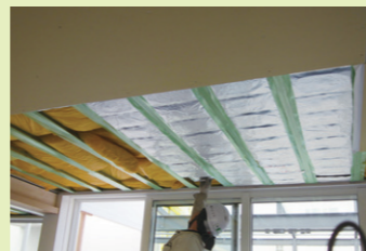
CALGRIP™ being installed on the ceiling
