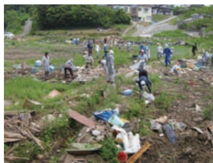
Our group's volunteer staff making rafts and removing debris
