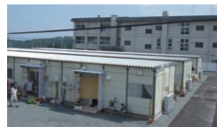
Temporary housing on Oshima, Kesennuma City
